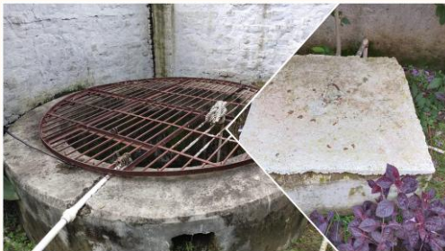
Water Management-Bore Well
